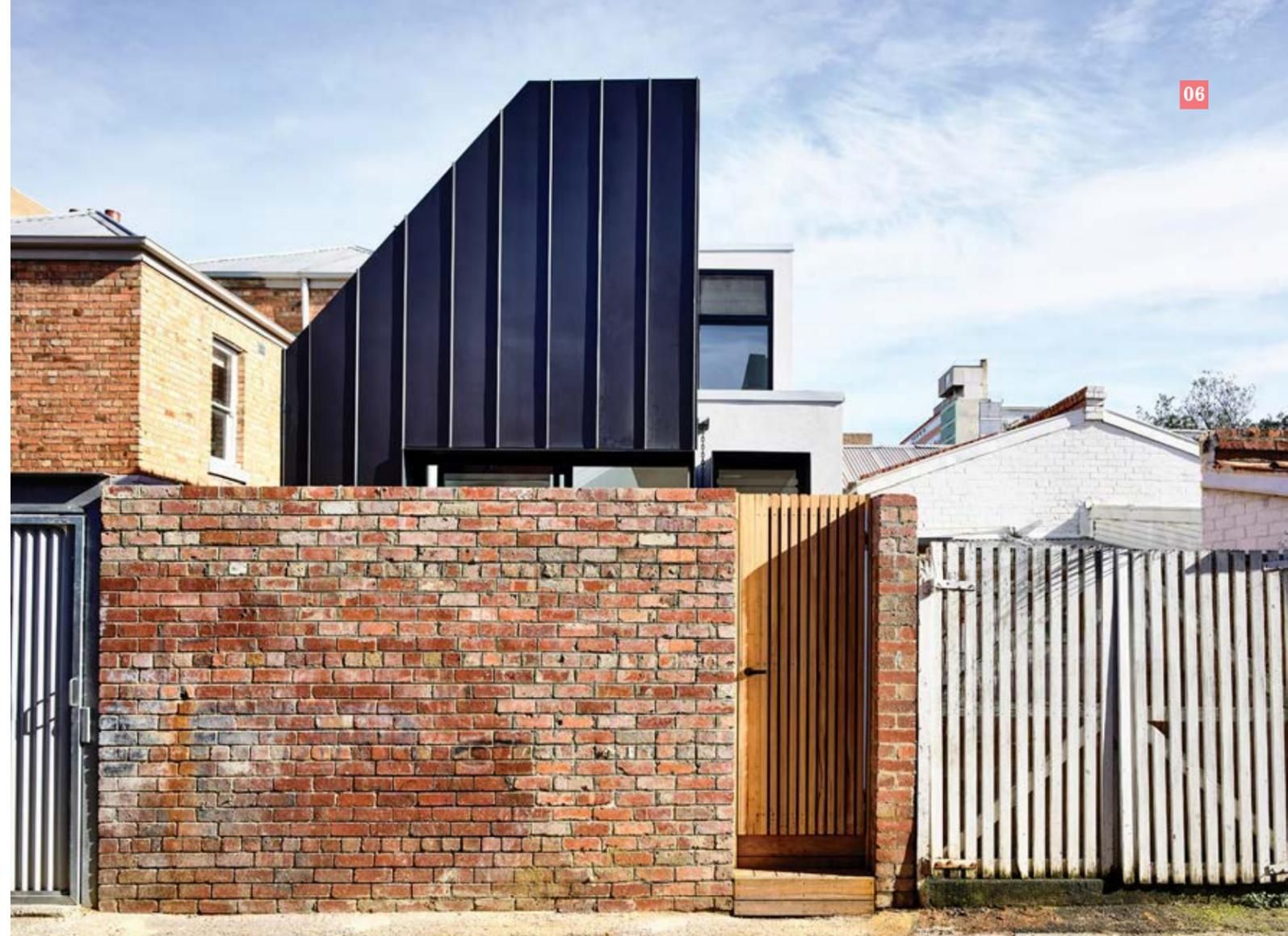
**06** The new eastern facade is clad in dark zinc panels and is set back from the laneway boundary to allow for a small courtyard.
